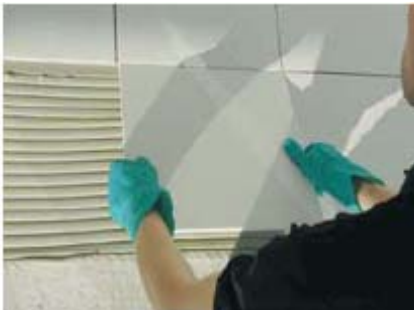
PCI Nanoflott flex can be applied as pourable bed adhesive as well as regular thin-bed adhesive.
