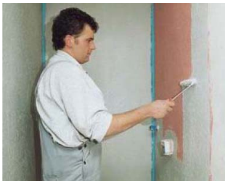
Application of undiluted PCI Lastogum to the substrate by roller, brush or trowel.
