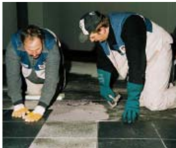
Natural stone coverings can be securely laid in the medium-bed method with PCI Carrament.
