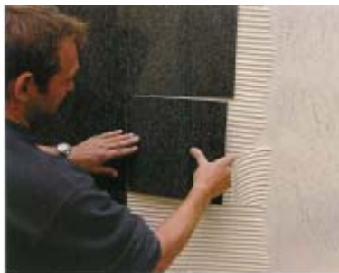
Laying of natural stone tiles on walls with PCI Carralight.
